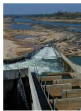
Pak Mun, Thailand (pool and weir type)
